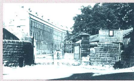
The Tannery before demolition.
